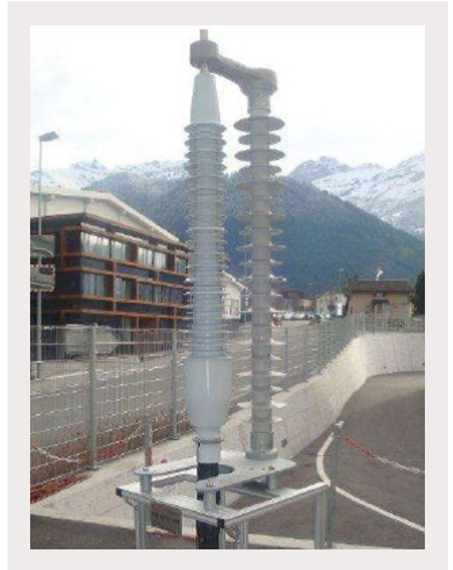
Fig. 3: Dry outdoor termination for substation application
