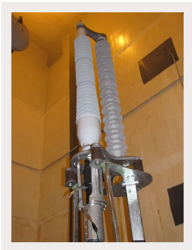
Fig. 6: HV cable termination type EST170-C53L during salt fog withstand
